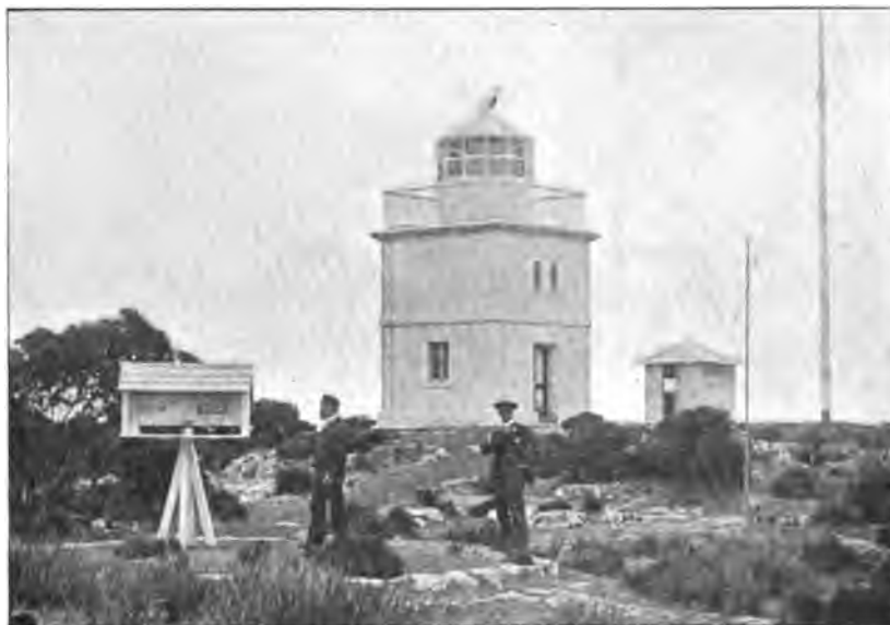
LIGHTHOUSE AND SIGNALLING STATION, CAPE BORDA.
